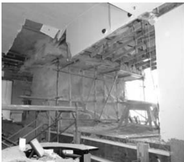
Overall View of Repair Using Shotcrete
